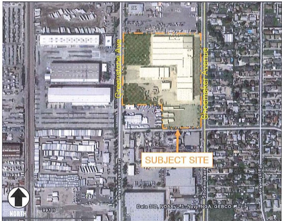
AERIAL PHOTOGRAPH – 11688 Greenstone Avenue
